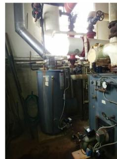
MES-M3 Oil-Fired Water Heater and Steam-to-Water Shell-and-Tube Converter
