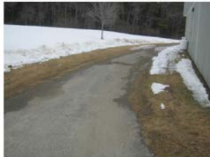
MHS-C7 Perimeter road around west side of school
