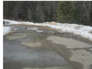
MHS-C8 Perimeter road at north side of building
