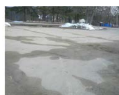
WES-C2 Pavements at entrance and Parking.
