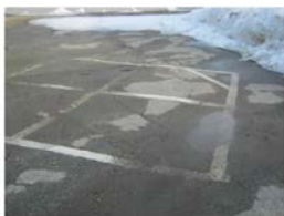
WES-C3 Pavement at west side of building.
