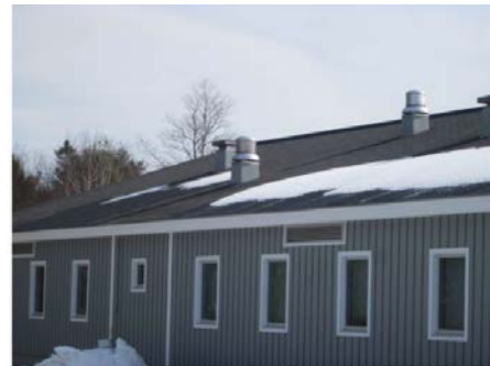
MHS-A8: Typical asphalt shingle roof system.
